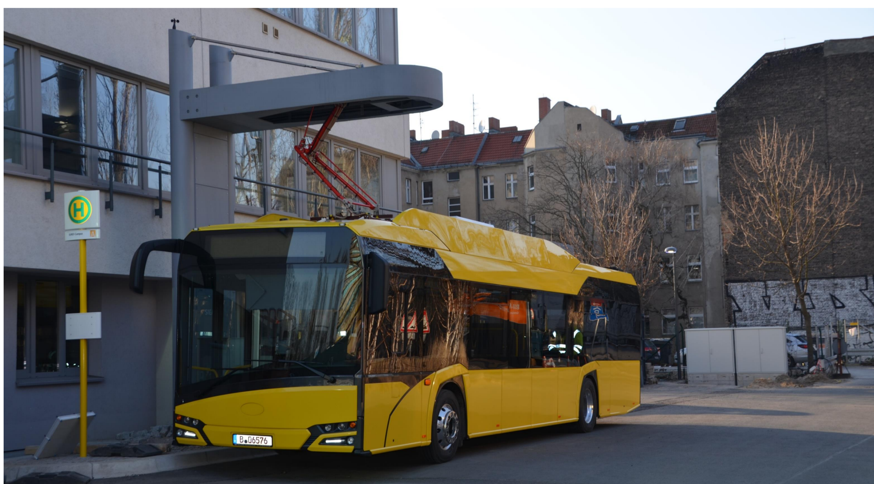
Fig. 1: Bus stop with charging station
